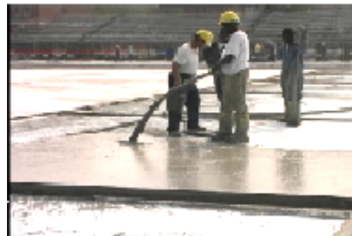
2. Lightweight Cement Poured on top of the roof from ground
