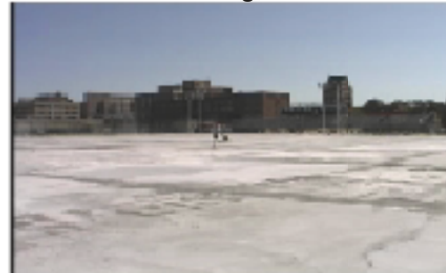
3. Hardening of Foamed Cement (140,000 square feet, 35 pcf, 300 psi)
